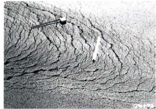
Figure 3. Irregular Crack
