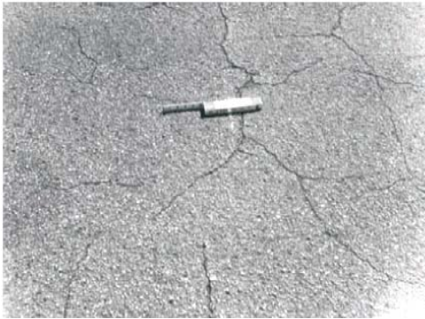
Figure 1. Block Crack
