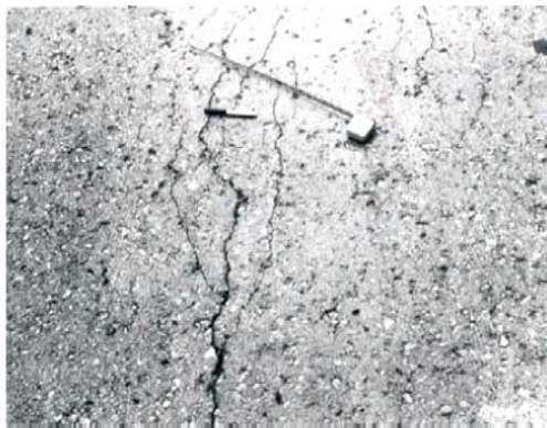
Figure 2. Alligator Crack
