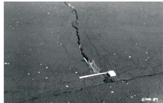
Figure 4. Transverse Crack
